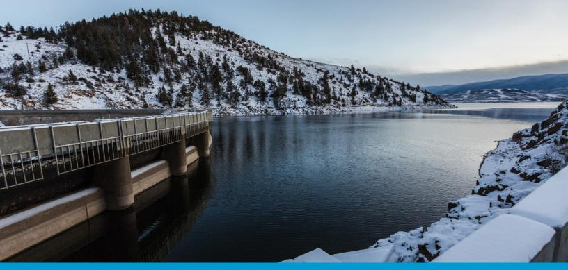
Completed in 1959, Williams Fork Dam & Power Plant sends water and electricity to the West Slope when Denver diverts water to the city. The dam backs up a reservoir that can store nearly 97,000 acre-feet of water.
